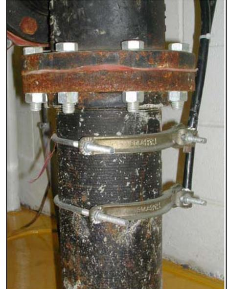
This sprinkler riser is appropriately bonded to the metal building in which it is located.
